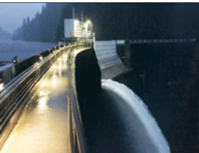
Our regional power wholesaler raised the water level at Swan Lake with an innovative addition to the dam—increasing hydro generating capacity by 25 percent.
