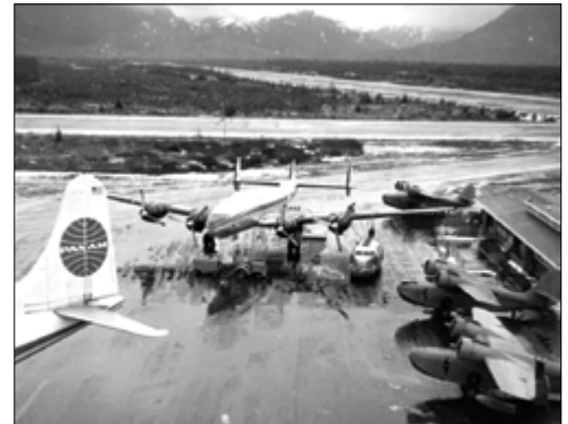
The WW II-era airport on Annette Island is left behind as Ketchikan International Airport opens in 1973. This photo depicts the Annette airport in its heyday, when Grumman Goose amphibians operated by Ellis Air Lines shuttled Ketchikan passengers to meet PanAm flights.
